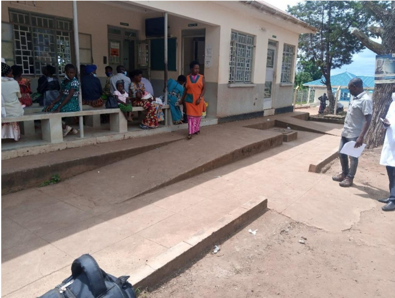
Figure 18:An example of a good continuous ramp linking different sections of the facility. (right)
