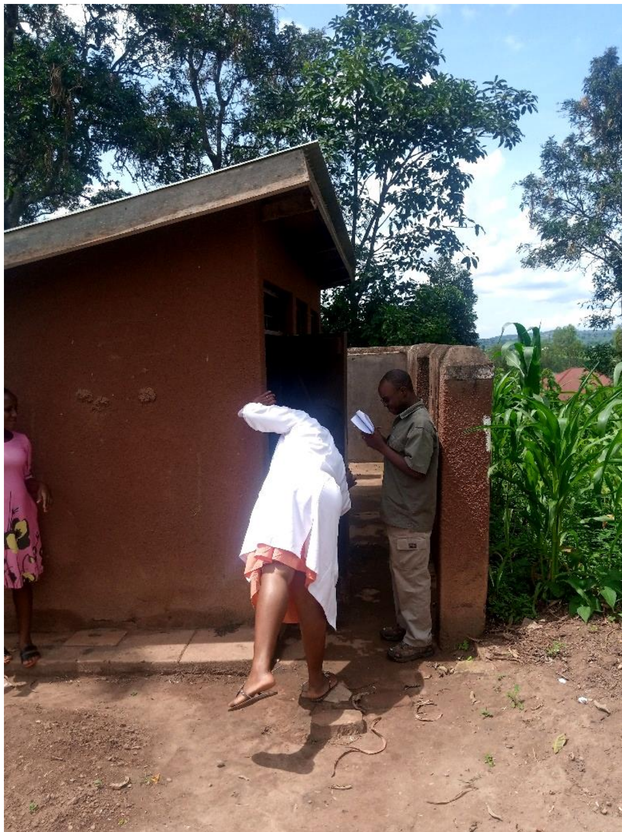
Figure 2: An example of inaccessible latrine outhouse
