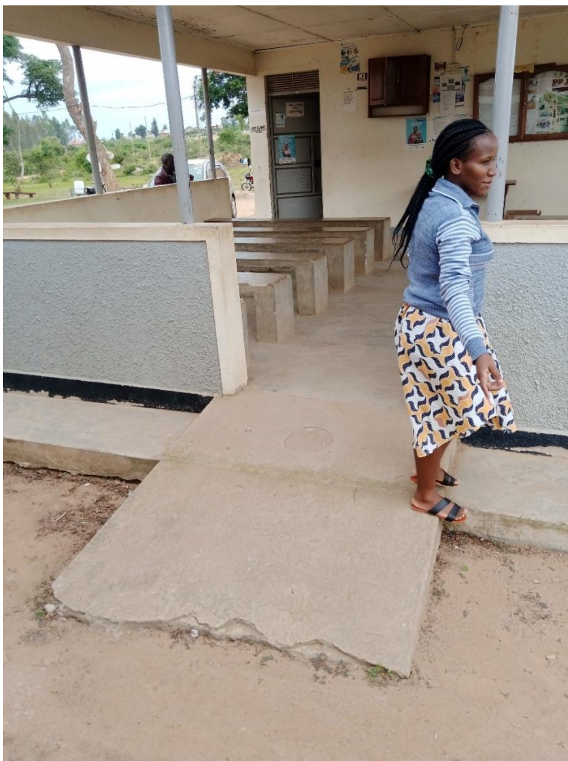
Figure 15: An example of a well-constructed ramp.
