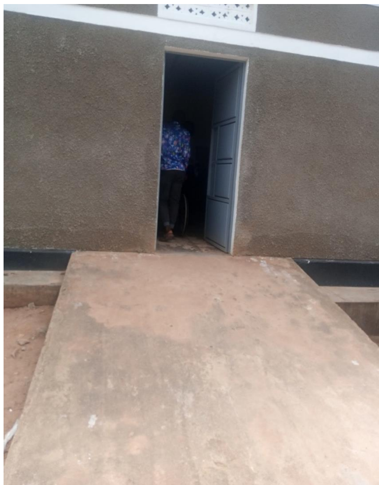
Figure 8: Ramp at the pharmacy
